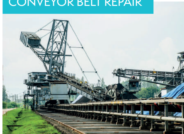
CONVEYOR BELT REPAIR
